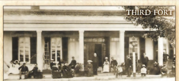
THIRD FORT To save money and quickly complete construction, buildings at the third fort were made of adobe and materials from the second fort.
